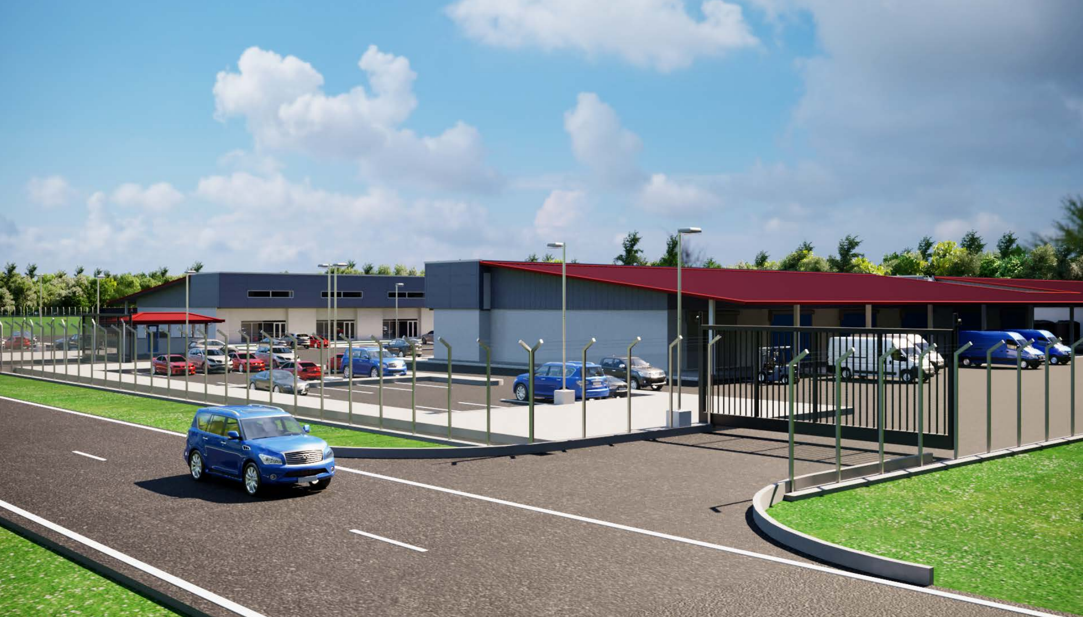
Warehouse Access Area
